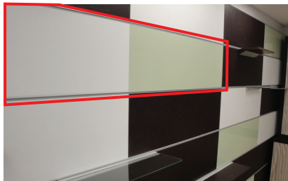
Snap in panels installed
