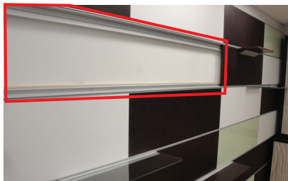
Snap in panels removed
